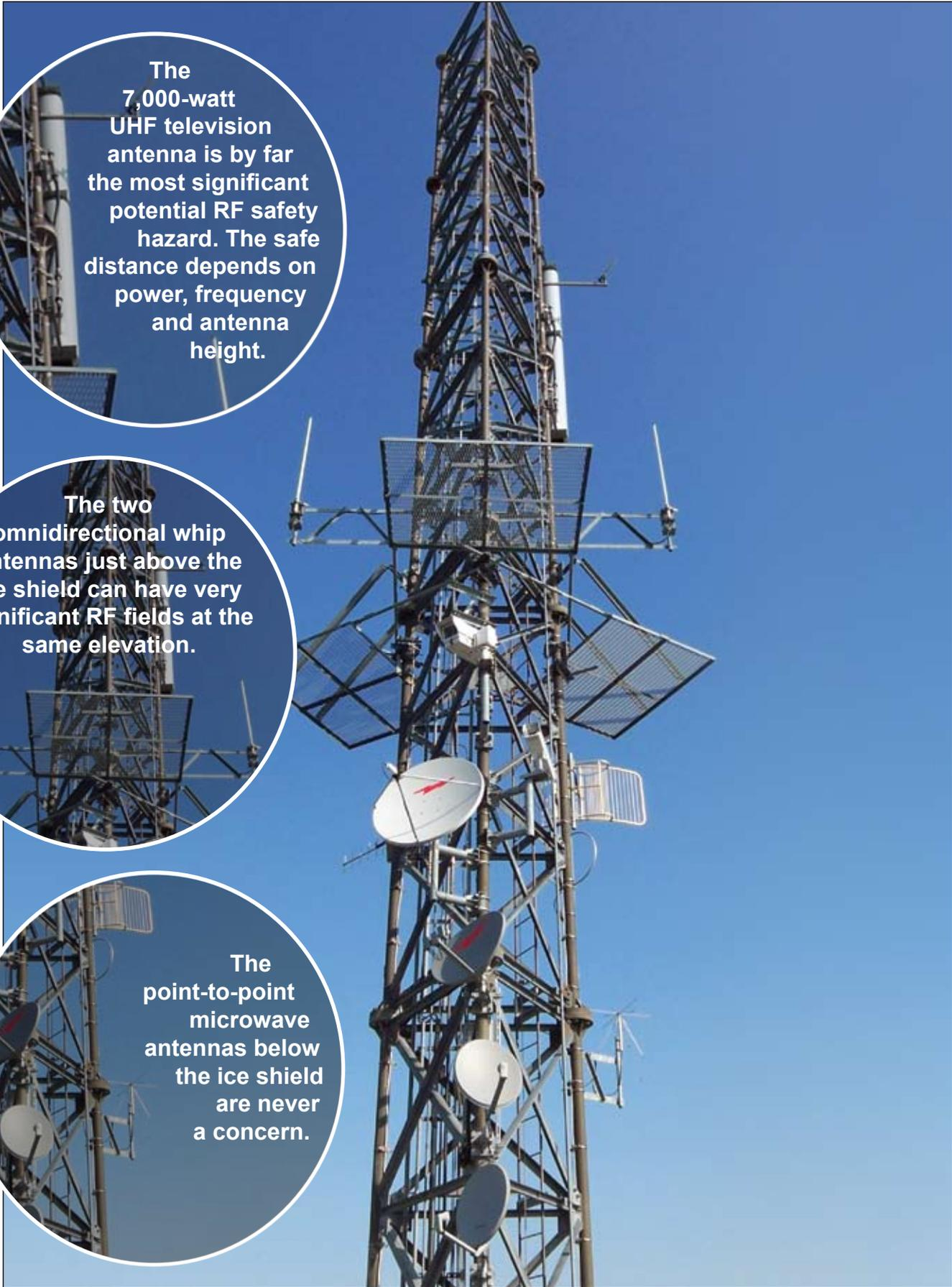
The 7,000-watt UHF television antenna is by far the most significant potential RF safety hazard. The safe distance depends on power, frequency and antenna height.
